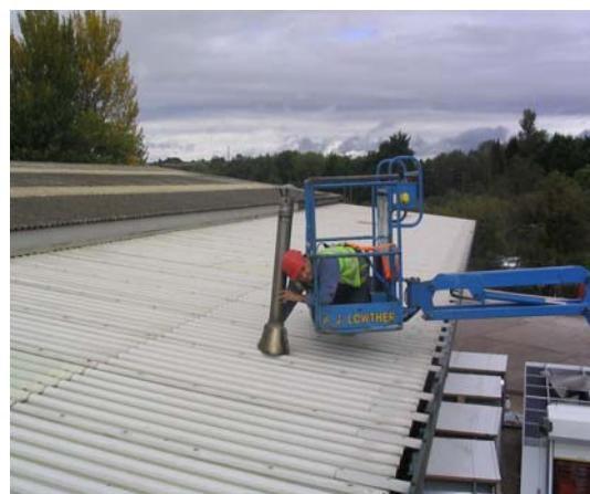
Figure 3 Using a MEWP to inspect a vent
