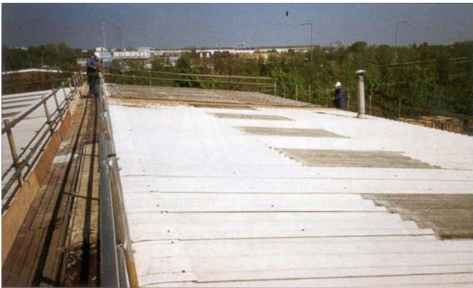
Figure 12 Complete overlidding of an AC roof
