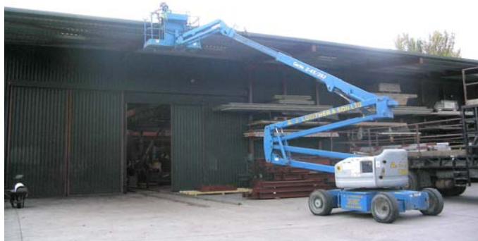
Figure 5 Using a MEWP to clean the gutter
