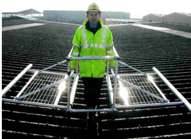
Figure 2 A personal fall prevention system
