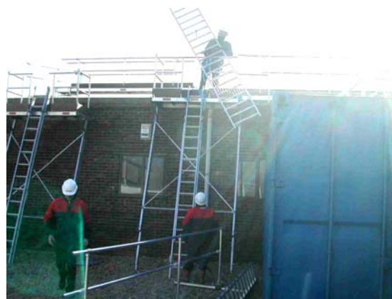
Figure 4 Installing a proprietary edge protection system
