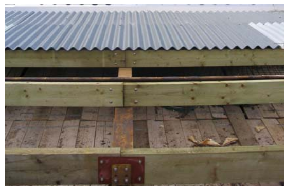
Figure 7 A crash deck providing collective fall protection
